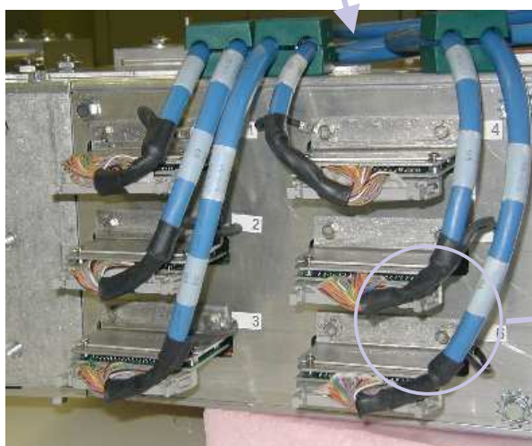
Fig.3a. Cable arrangement at the AFEB's output. All cables must go along the connector side wall.
